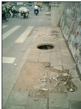
figure 26: bad surface of sidewalks on the western roadside
