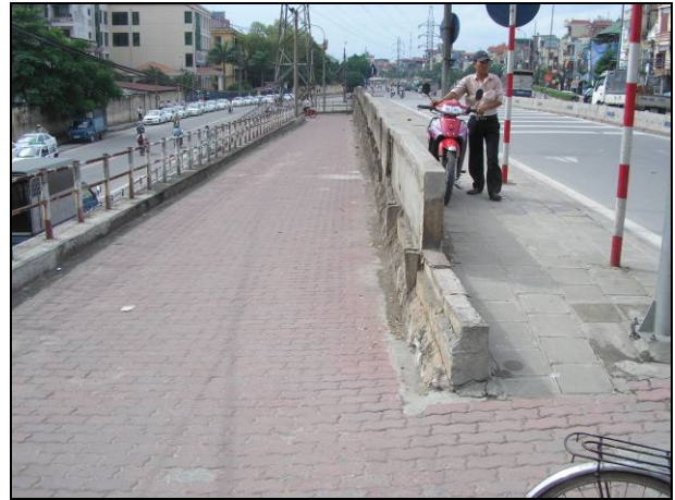
figure 16: bicycle ramp to allow crossing the central reservation
