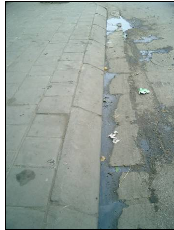
figure 22: flattened curbstones
