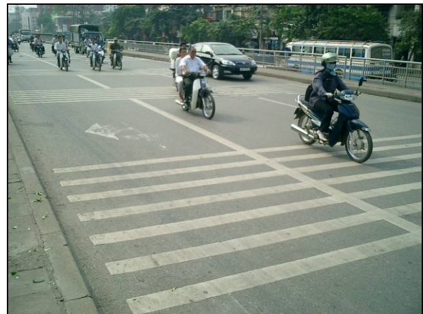
figure 20: ineffective speed-reducing measures
