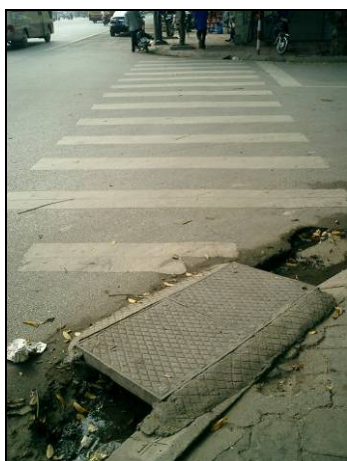
figure 27: steel ramps at pedestrian crossings
